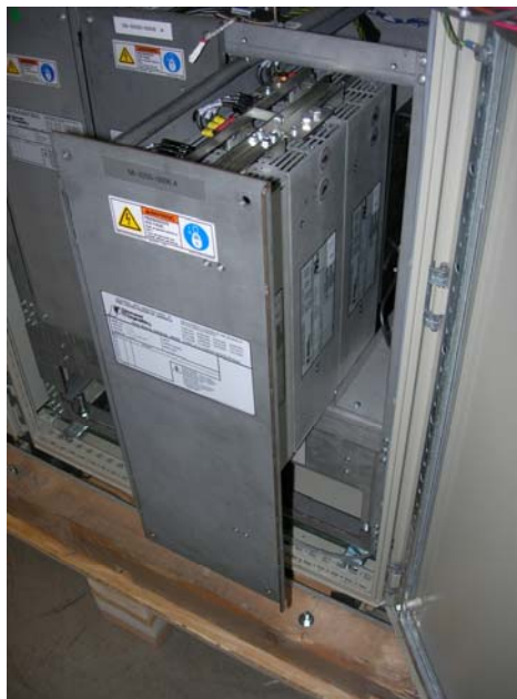
Figure 35 Sliding the Power Supply Module into the Frame
