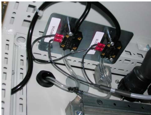
Figure 10 Pressure Switches (PSW121 A&B)
