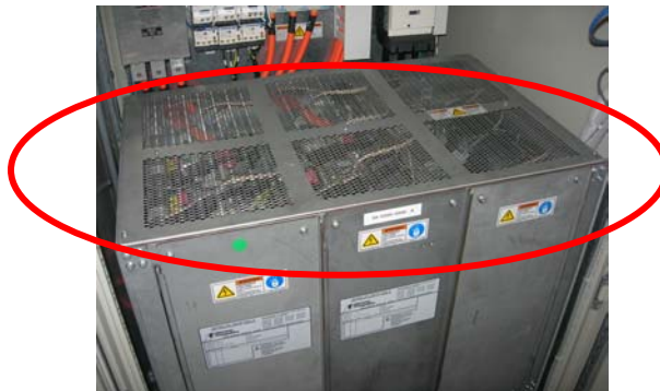
Figure 23 Power Supply Frame Top Screen
