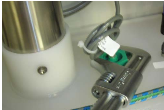
Figure 55 Removing the Old Level Sensor (LS201)
