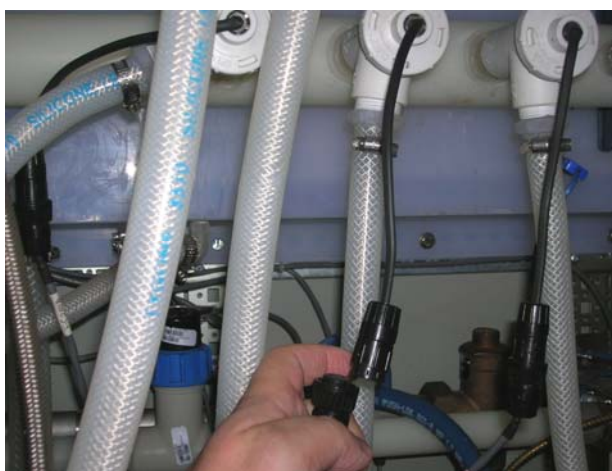
Figure 47 Unplugging the Flow Switch
